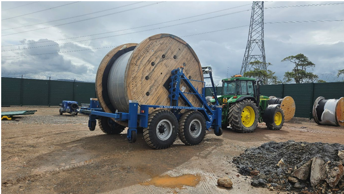
275kV cable ready to installed through ducting to connect the project to Scottish Power's substation.
