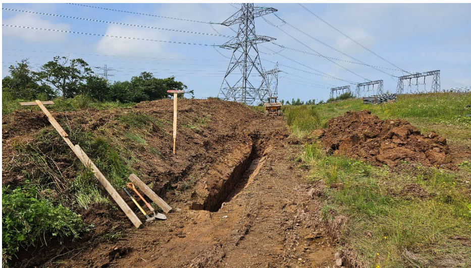
Trenches for cables connecting the project to the substation
