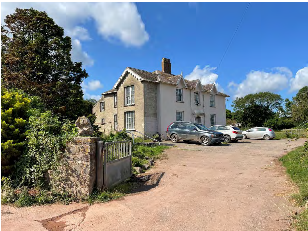
Plate 10: Close-ranging view of Alleston Farmhouse (east- and north-facing elevations) from its driveway
