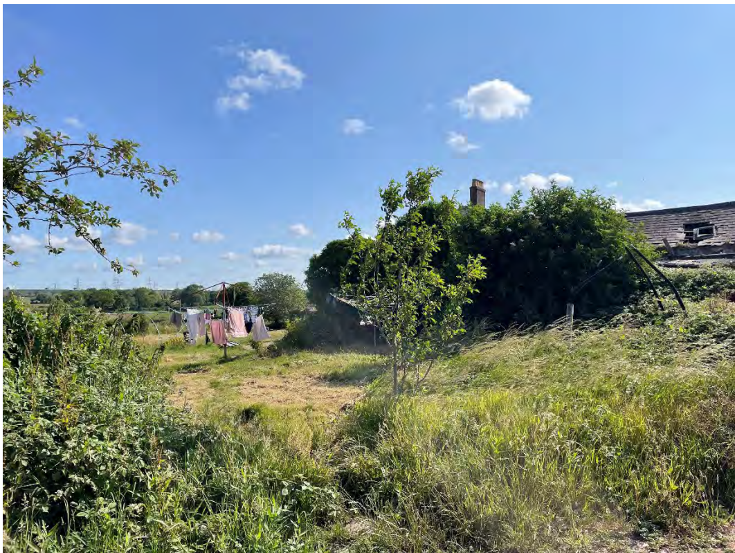
Plate 12: Very limited visibility of Alleston Farmhouse from the section of farm track to the south-west; only its chimney and part of the attached outbuilding are visible
