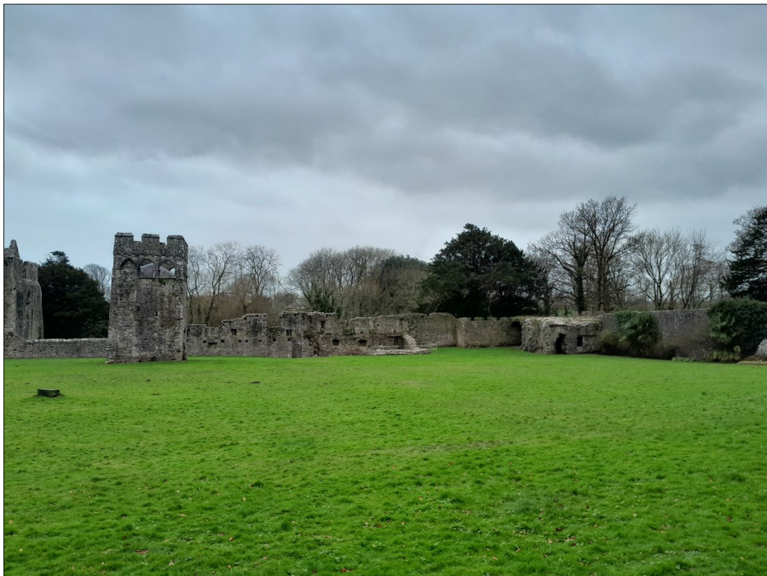
Plate 17: View north-east across the Bishops Palace Scheduled Monument (PE003) and Grade I Listed Building (17393), view towards the Site
