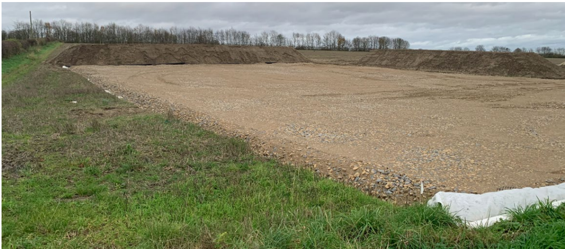
Insert 15: Newly laid Construction Compound (Elsham-Lincoln Pipeline)
