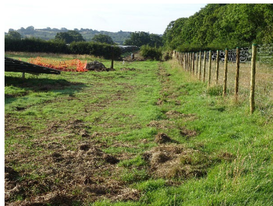
Insert 63: Topsoil Replaced
