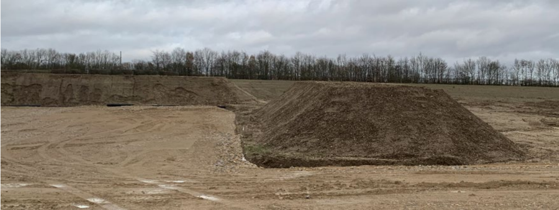
Insert 17: Topsoil Storage Bund (example from Lincolnshire)
