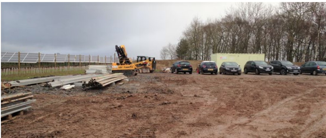
Insert 20: Start of Restoration of Construction Compound (example from Staffordshire)
