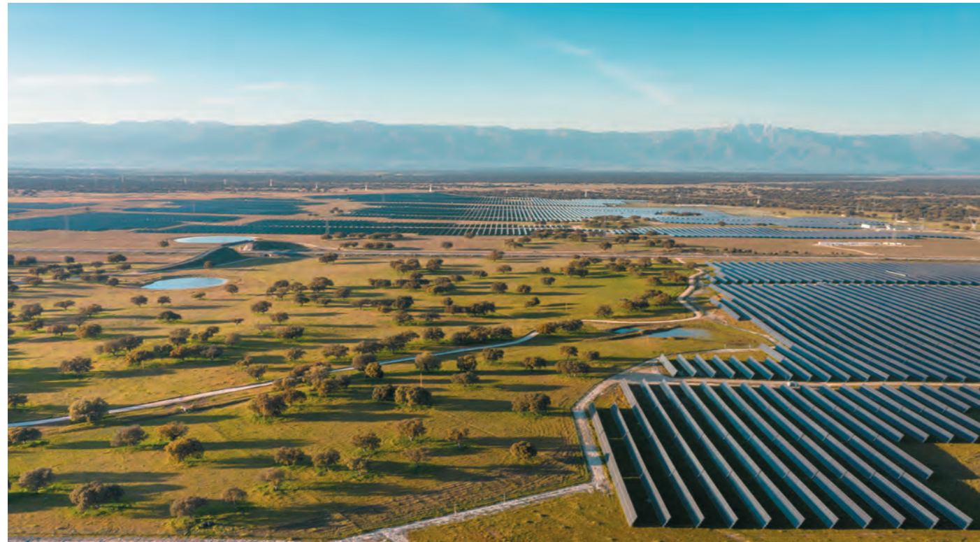
Statkraft’s Talayuela Solar Farm, Spain
