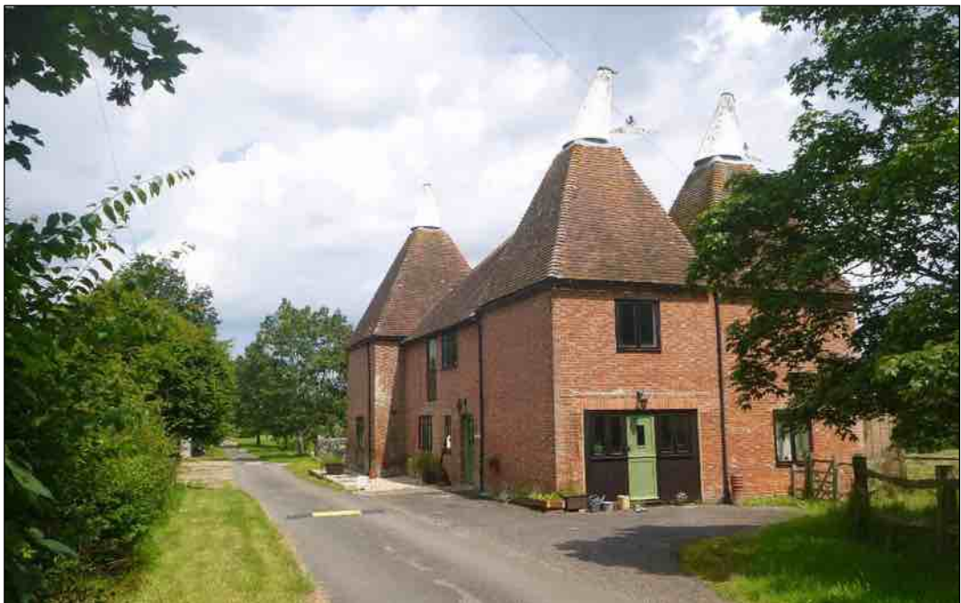
Photo. 6 Oasthouse 60m north-east of Little Cheveney Farm, looking north
