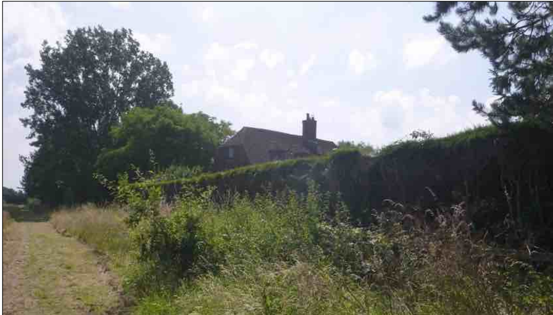
Photo. 15 Limited views of Turkey Farm House from adjacent footpath, looking south-east
