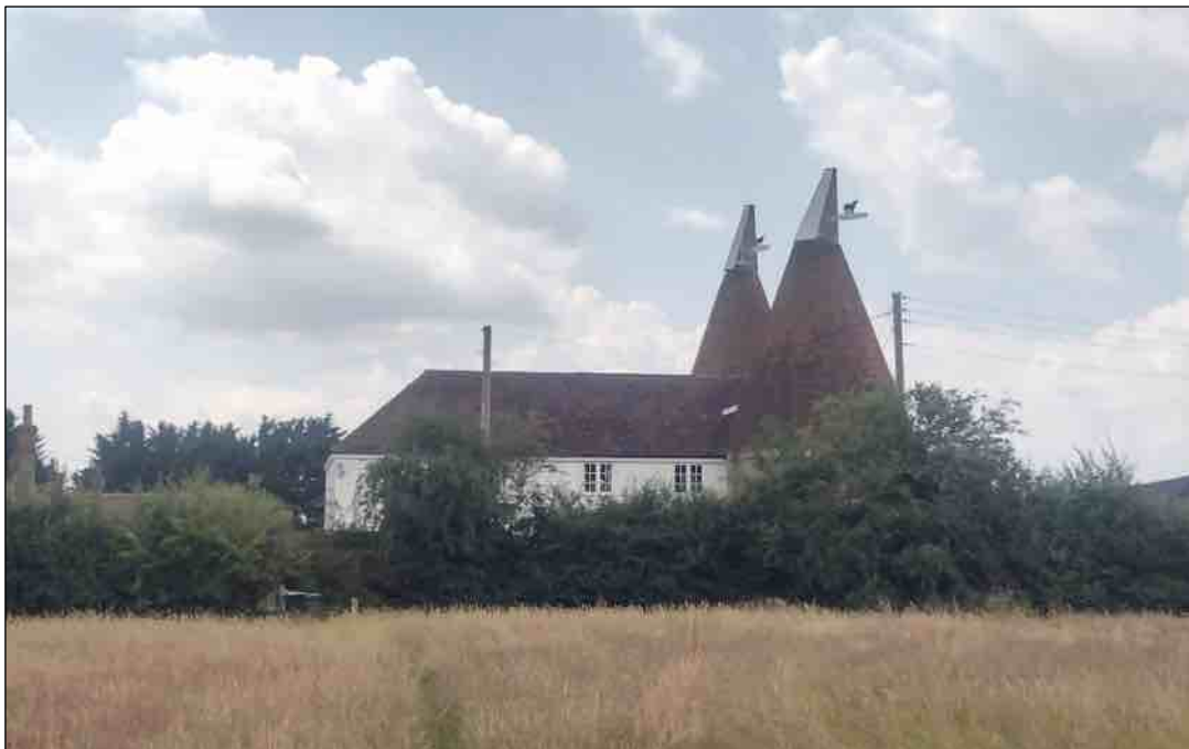
Photo. 13 View of Great Sheephurst Oasthouse from footpath, looking south-west
