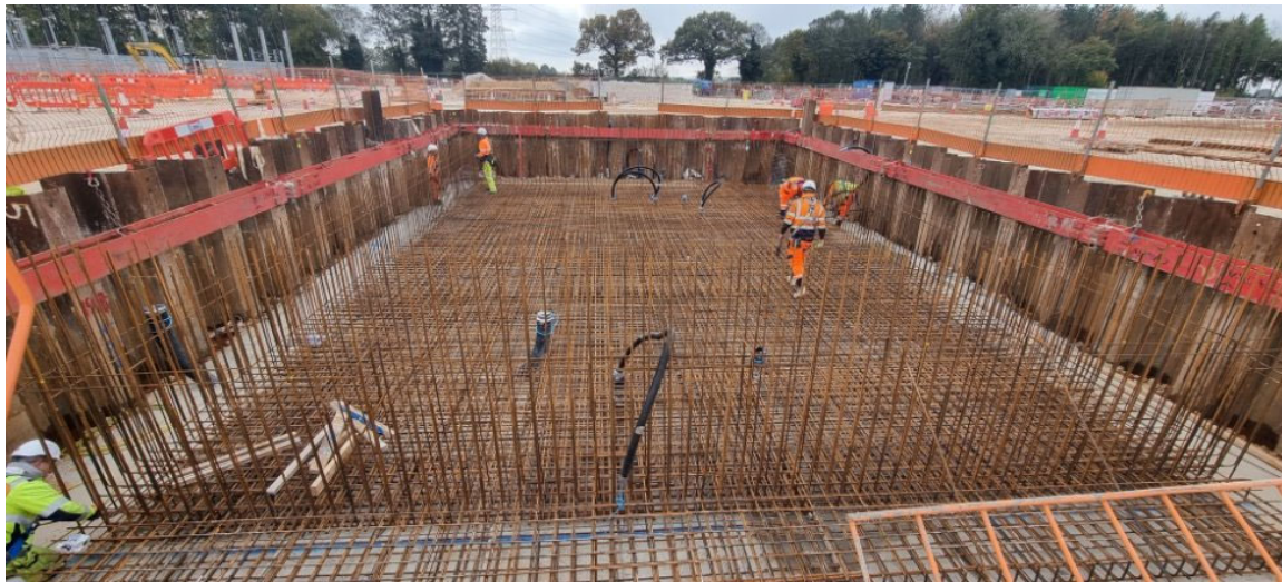
Steel Reinforcement for Main Transformer Base 24/10/2024
