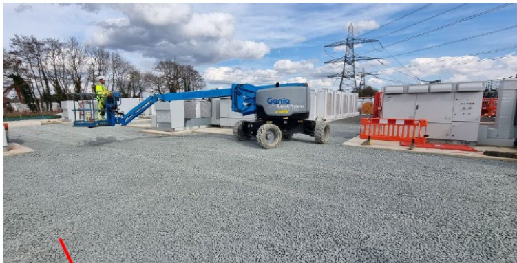
Stoning up between the cubes in Collector 1 27/03/25.
