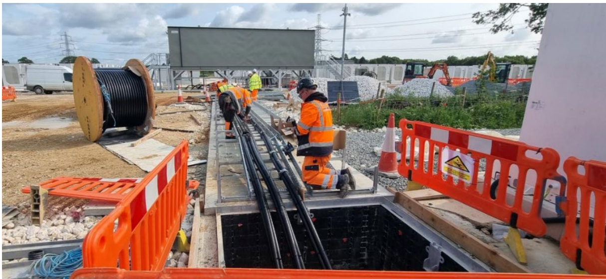
Cable pulling between the switchboard and switchgear building, June 2025
