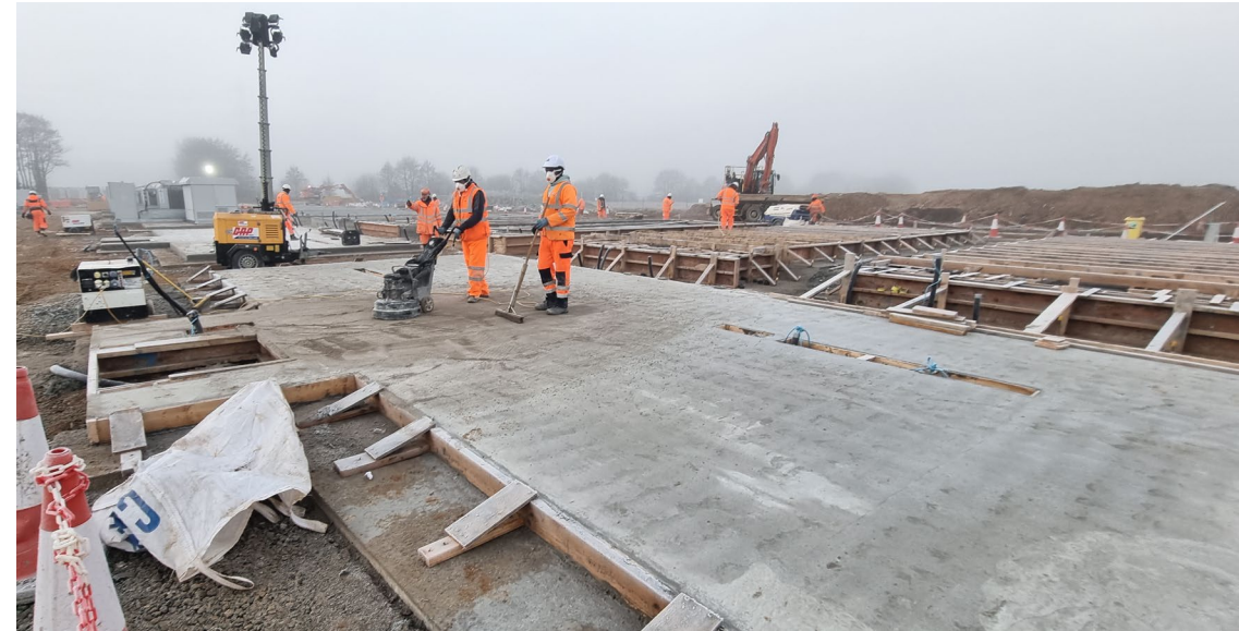
Team working on the Twin Skid Foundations 16/01/2025
