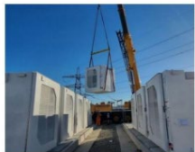
Battery units being installed on site
