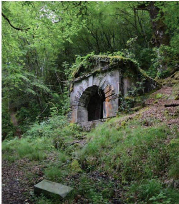
Note deterioration of structure, vegetation ingress, and fallen stonework.
