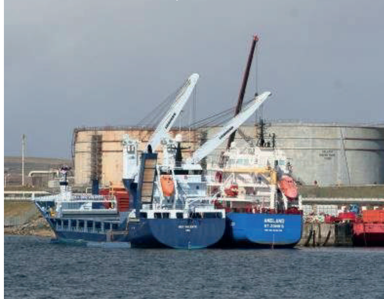
Sullom Voe Construction Jetty
