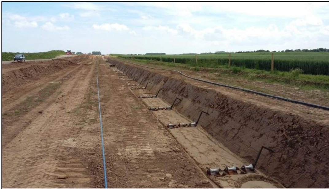
Plate 2-3: Typical UGC Trench
