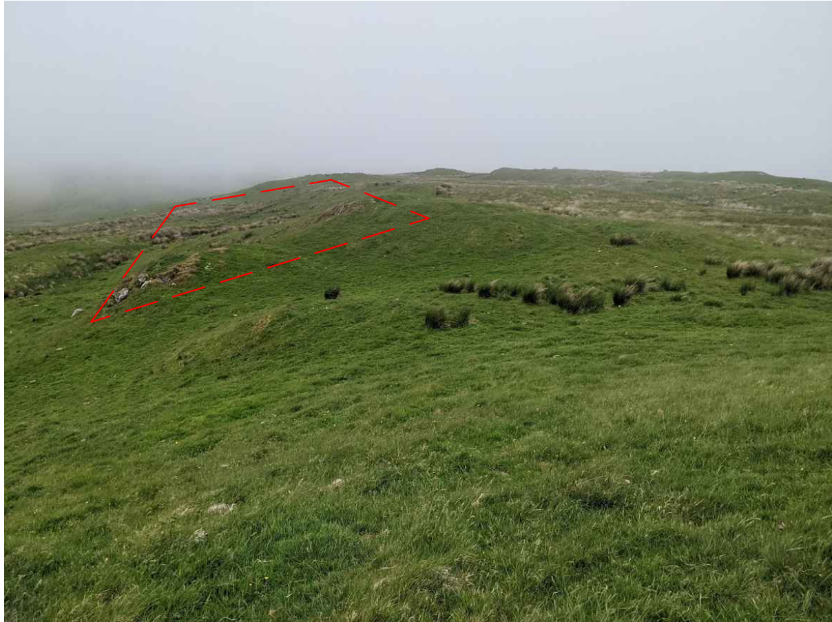
Borrow Pit C Approximate location marked with red dash. Steeply sloping ground and rock outcropping at the surface observed at this location. Photograph taken from east side of borrow pit.
