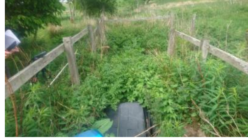
Fenced off area around collection tank
