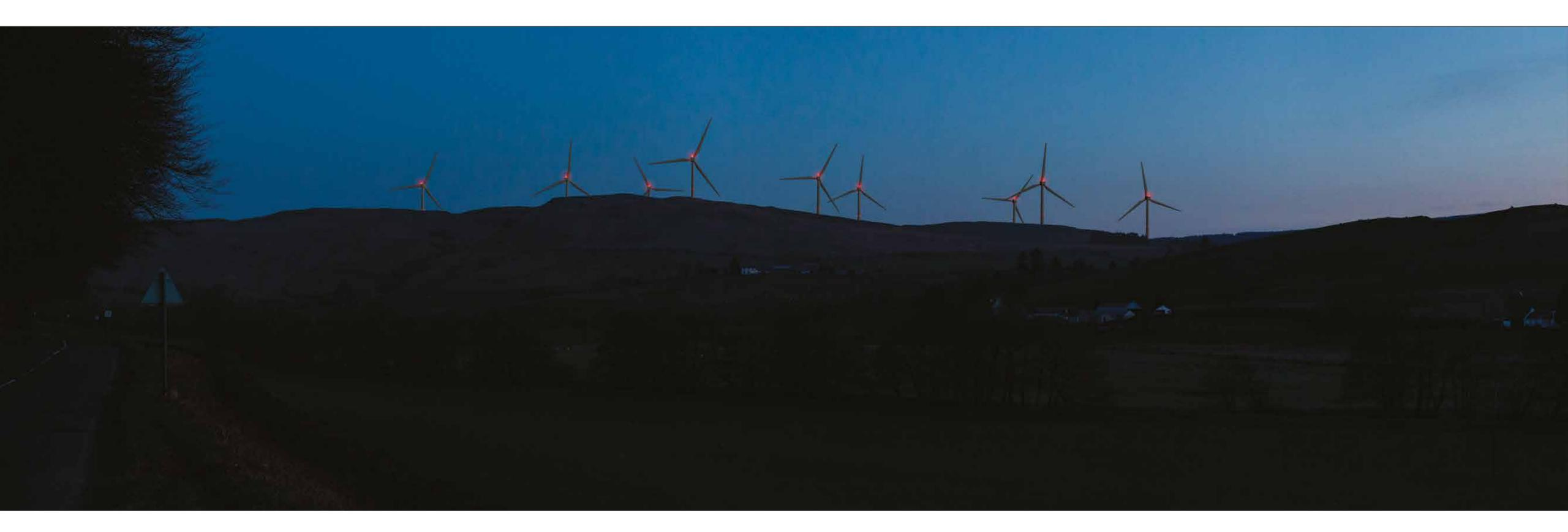
Photomontage showing submission layou 9 turbines: 6 @ 200m to blade tip height and 3@180m to blade tip height. All turbines shown with a 155m rotor diameter. Note: Turbines over 150m are required to be fitted with lighting and required to be lit to the equivalent of 200 candela, taking into account the prevailing weather conditions, when light fades.
