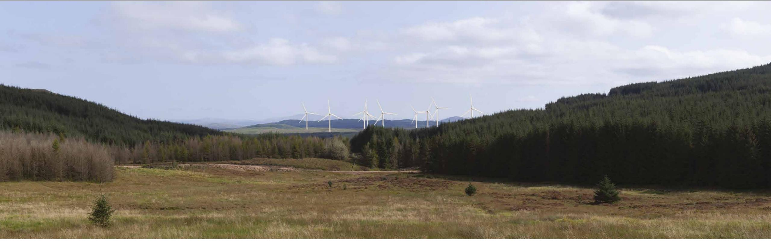
Photomontage showing submission layout 9 turbines: 6 @ 200m to blade tip height and 3@180m to blade tip height. All turbines shown with a 155m rotor diameter.
