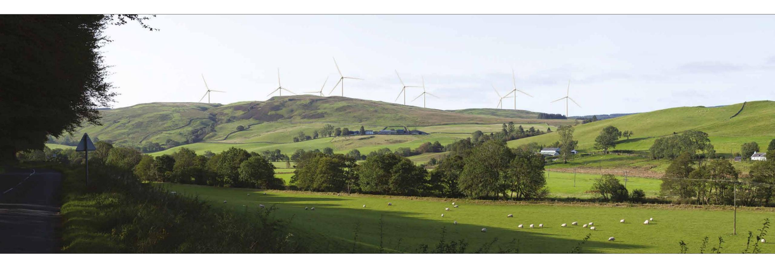
Photomontage showing submission layout 9 turbines: 6 @ 200m to blade tip height and 3@180m to blade tip height. All turbines shown with a 155m rotor diameter.
