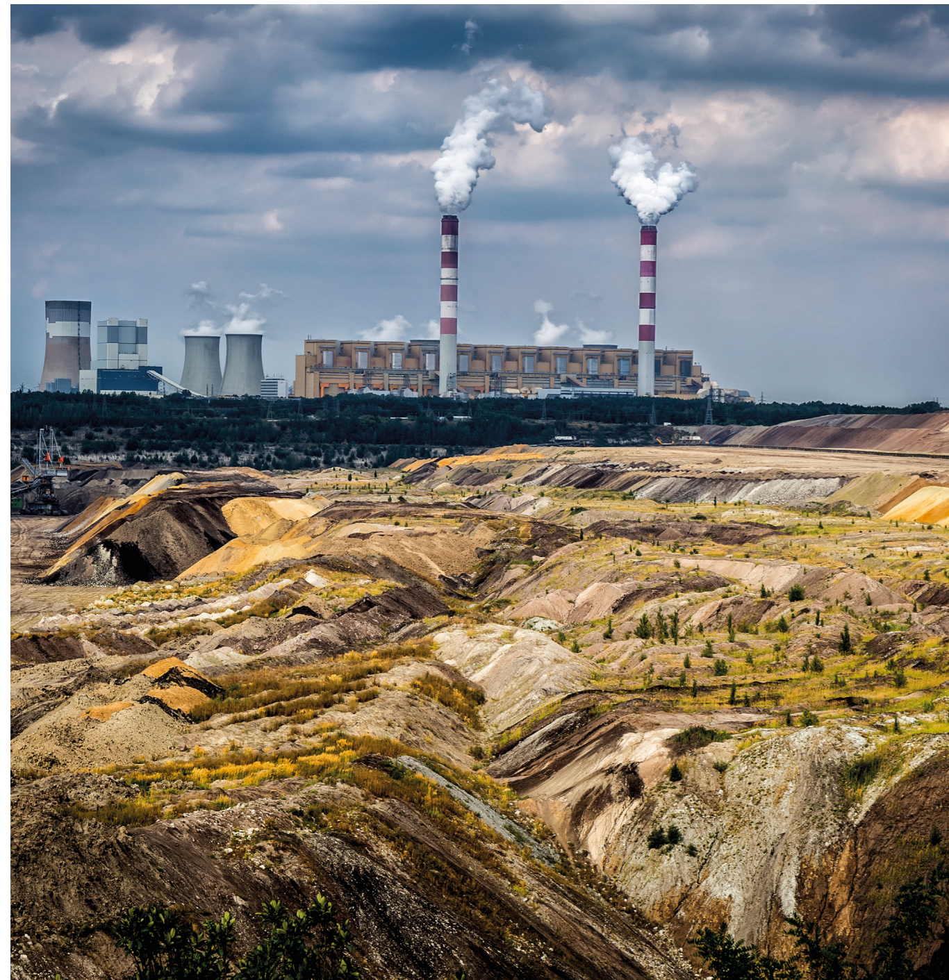
COAL POWER PLANT in the city of Bełchatów, Poland
