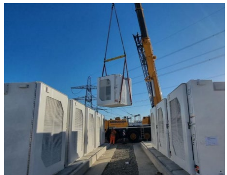
Battery units being installed on site
