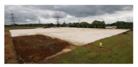
Replacing topsoil with crushed stone to support the battery foundations. Temporary drainage systems including swales and attenuation ponds have been installed to control surface water runoff rates during construction.
